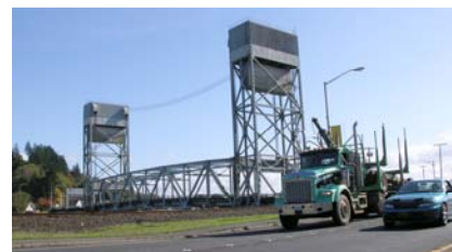
Riverside Avenue Bridge
