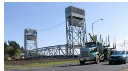
Riverside Avenue Bridge
