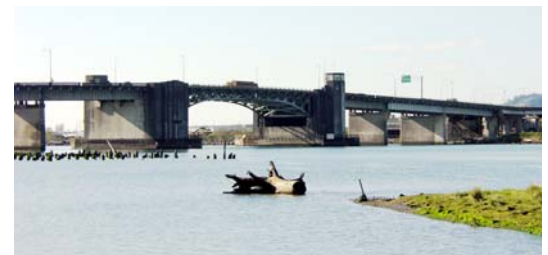
The Chehalis River Bridge provides access between South Aberdeen/Cosmopolis and US 12/downtown Aberdeen.
