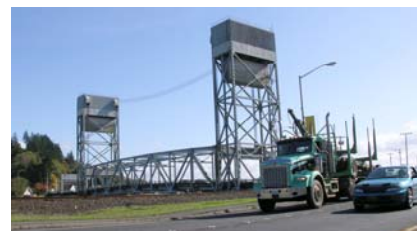
Riverside Avenue Bridge
