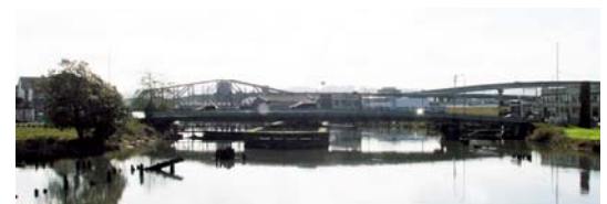
The Heron Street Bridge is an important link in the region's transportation network.
