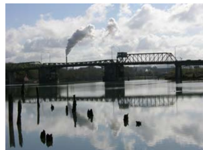
Simpson Avenue Bridge
