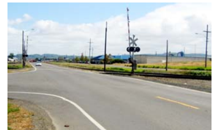
The two at-grade railroad crossings along Port Industrial Road would be removed in conjunction with this project.
