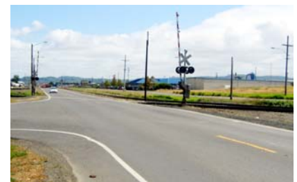
The two at-grade railroad crossings along Port Industrial Road would be removed in conjunction with this project.
