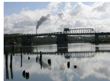
Simpson Avenue Bridge
